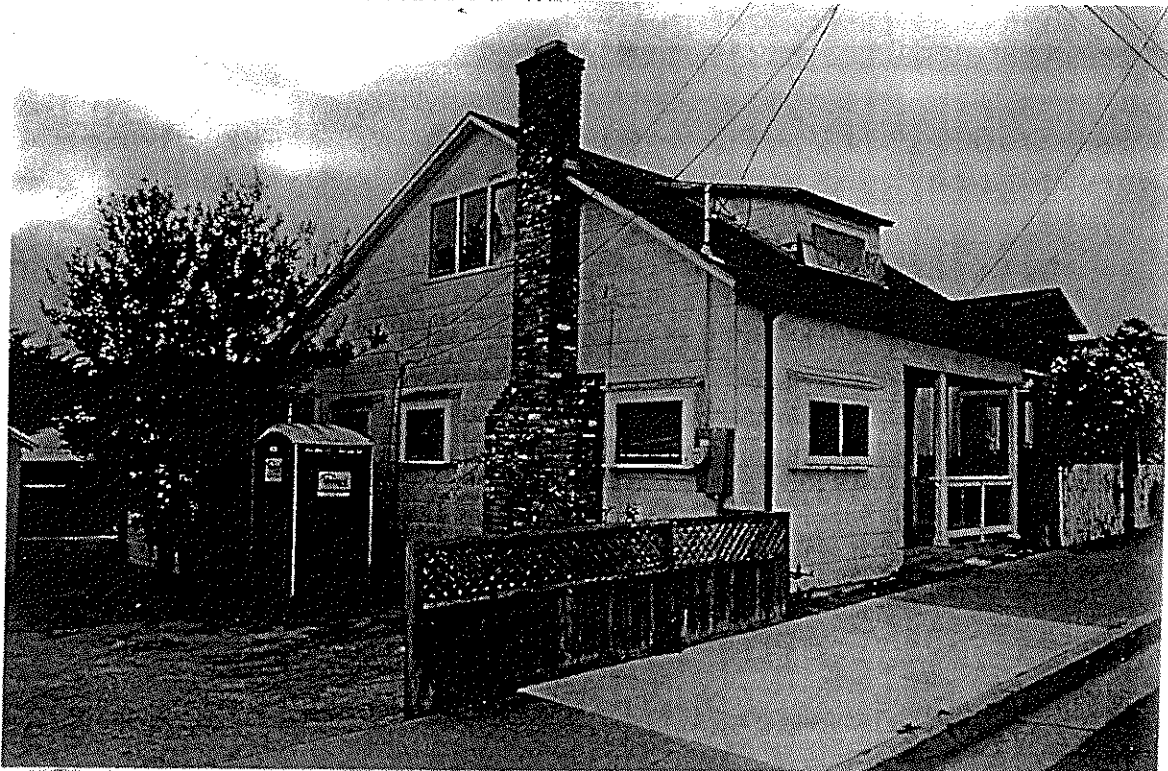
Photo #2. Looking SE at the north side & front elevations. August, 2014.
